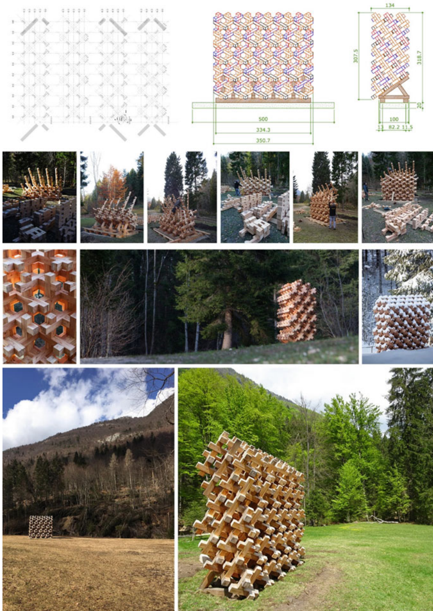
Fig. 2 Forest Byobu design definition ( drawings credit Galloppini Legnami and Politecnico di Milano) and assembling phases ( credit Politecnico di Milano), up to the final complete structure, a geometric pattern contrasting the natural landscape of its location at Arte Sella, the Contemporary Mountain ( credits for the first row, Ph. Giacomo Bianchi for Arte Sella; for the latter, Politecnico di Milano)
