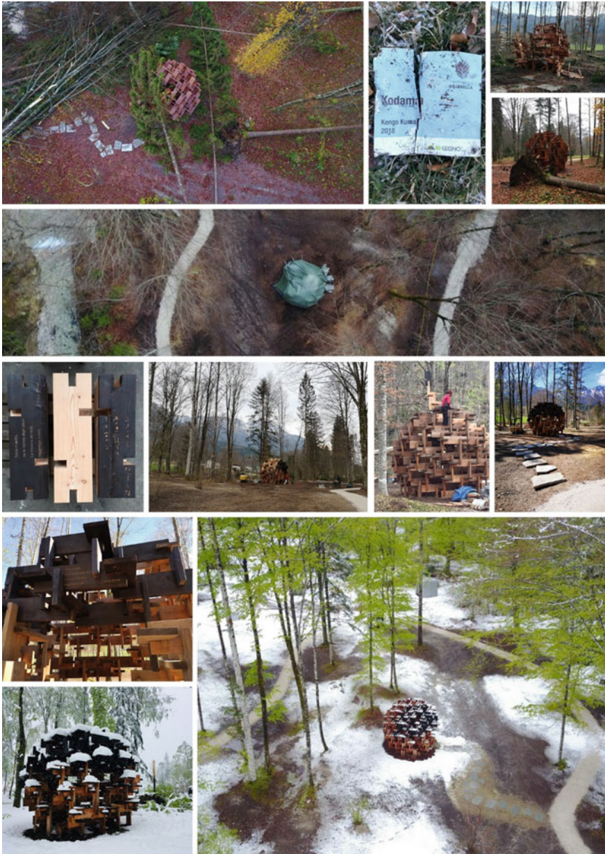
Fig. 6 Kodama 2.0 is the Arte Sella pavilion refurbishment damaged during the devastating storm of October 2018: the structure has been (i) protected to retain the humidity content of wood elements before restoration; (ii) new pieces have been cut via CNC machine, (iii) burned and carved to render a Japanese haiku on the surface, and (iv) relocated to its original location, obtaining a new aesthetic for the wooden lattice ( credit Politecnico di Milano and Arte Sella)
