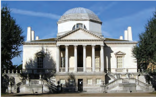
Figure 7.18 / Chiswick House, London
