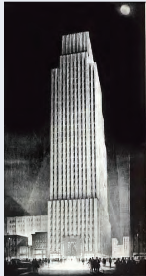
Figure 2.45 | New York Daily News Building
