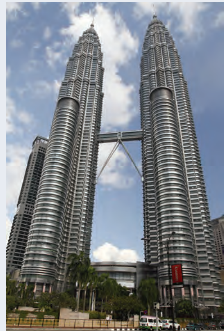
Figure 7.38 | Petronas Twin Towers, Malaysia
