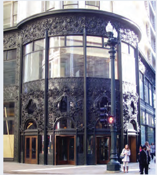
Figure 7.35 | The northwest entrance to the Carson, Pirie, Scott and Company Building
