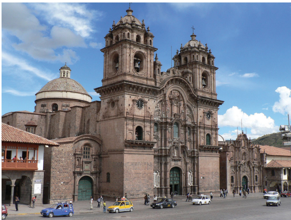
Figure 6.5: The Jesuit Church of La Compañía de Jesús on the Plaza de Armas in Cuzco, Peru The original church was constructed in 1571 on the site of the ancient Incan palace. The earthquake of 1650 caused severe damage to the building, so it had to be reconstructed in about 1688. Many Catholic cathedrals in Latin America were built with stones from ancient sites. This cathedral is claimed to be the Western Hemisphere’s most ideal example of colonial baroque architecture. James Preston – La Compania de Jesus, Cusco – CC BY 2.0.
