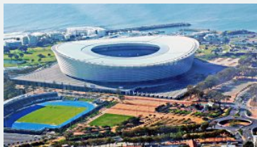
Figure 7.58 Cape Town Stadium, Taken from Signal Hill, South Africa; Seating Capacity of 64,100
