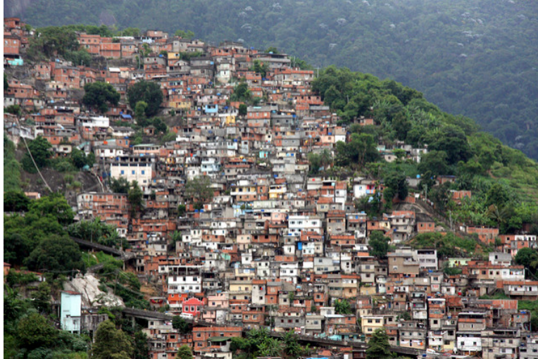
Figure 6.27: Favela La Rocinha, Rio de Janeiro, Brazil Favelas are usually self-constructed and start out as slums. Many lack ownership rights, police protection, or public services. With time, some become established neighborhoods. Pedro Lopez – Favela, Rio de Janeiro – CC BY 2.0.
