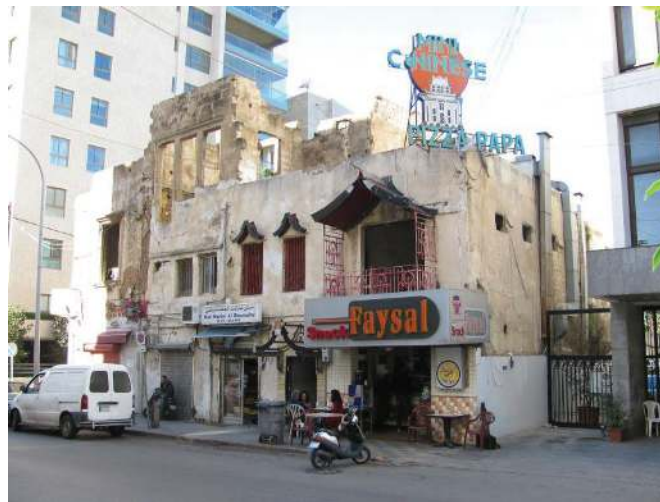
Figure 8.33: Beirut, Lebanon Located in the middle of an upscale neighborhood in Beirut, this food shop is in a building that has not been fully repaired from damage resulting from the 1975 civil war. The restaurant offers diverse foods, including Chinese food and pizza. Steven Damron – mini chinese , pizza papa , faysal – CC BY 2.0.
