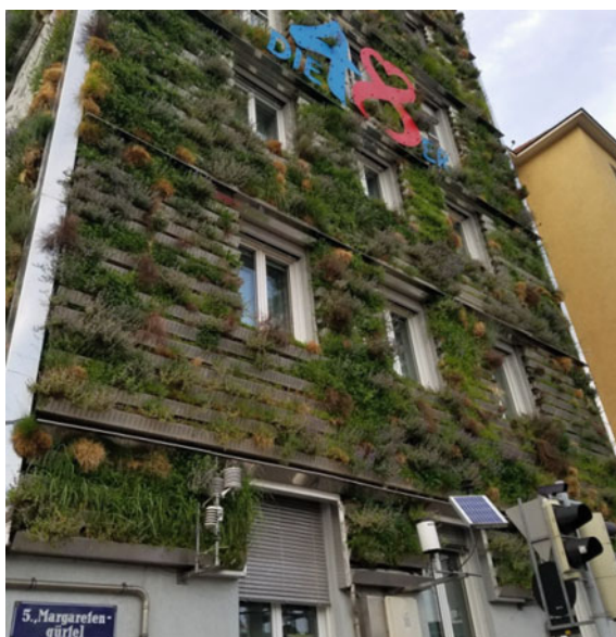
Fig. 1 “Climate façade” on the MA48 building, Vienna
