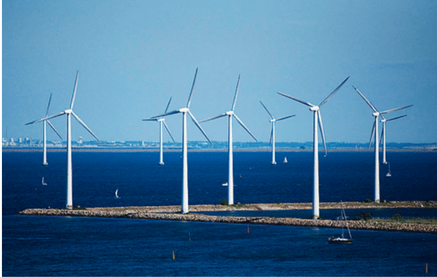
Wind farm near Copenhagen, Denmark. In 2014 wind power met 39% of electricity demand in Denmark.
