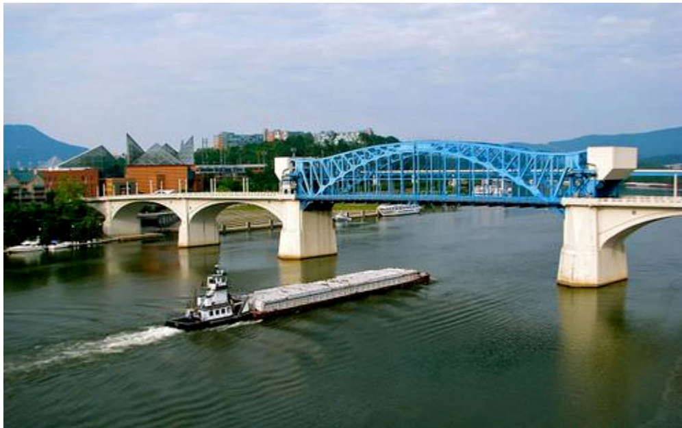
Figure 1. The John Ross Bridge, in Chattanooga, Tennessee.
