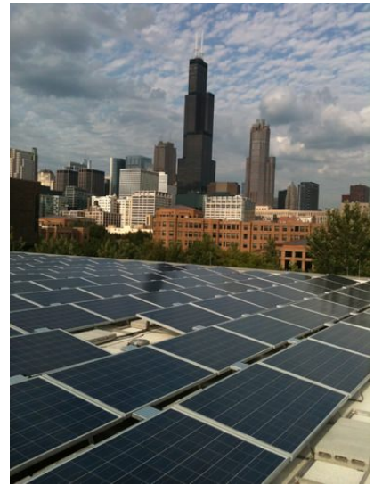
Figure 4. Rooftop Solar Installations Rooftop solar installation on Douglas Hall at the University of Illinois at Chicago does not affect land resources while producing electricity with zero emissions. Source: Office of Sustainability, UIC
