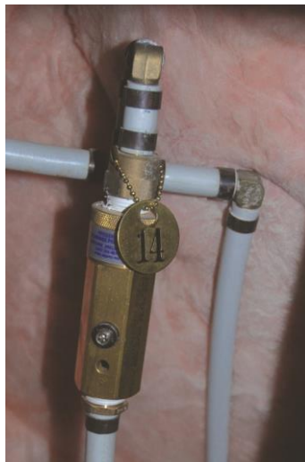
Figure 6-46—Trap primer NOT approved AG
