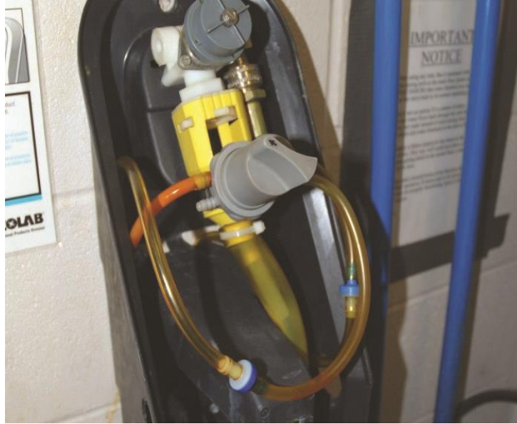
Figure 4-34—Air space vacuum breaker
