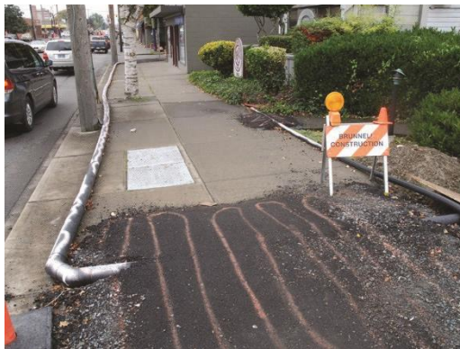
Figure 3-8—Temporary service connection completed above ground at the service connection
