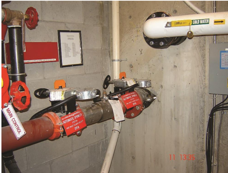
Figure 6-57—Fire sprinkler system class 1 no chemical additives
