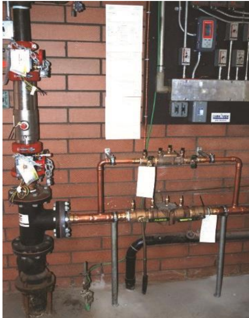
Figure 6-12—A parallel installation
