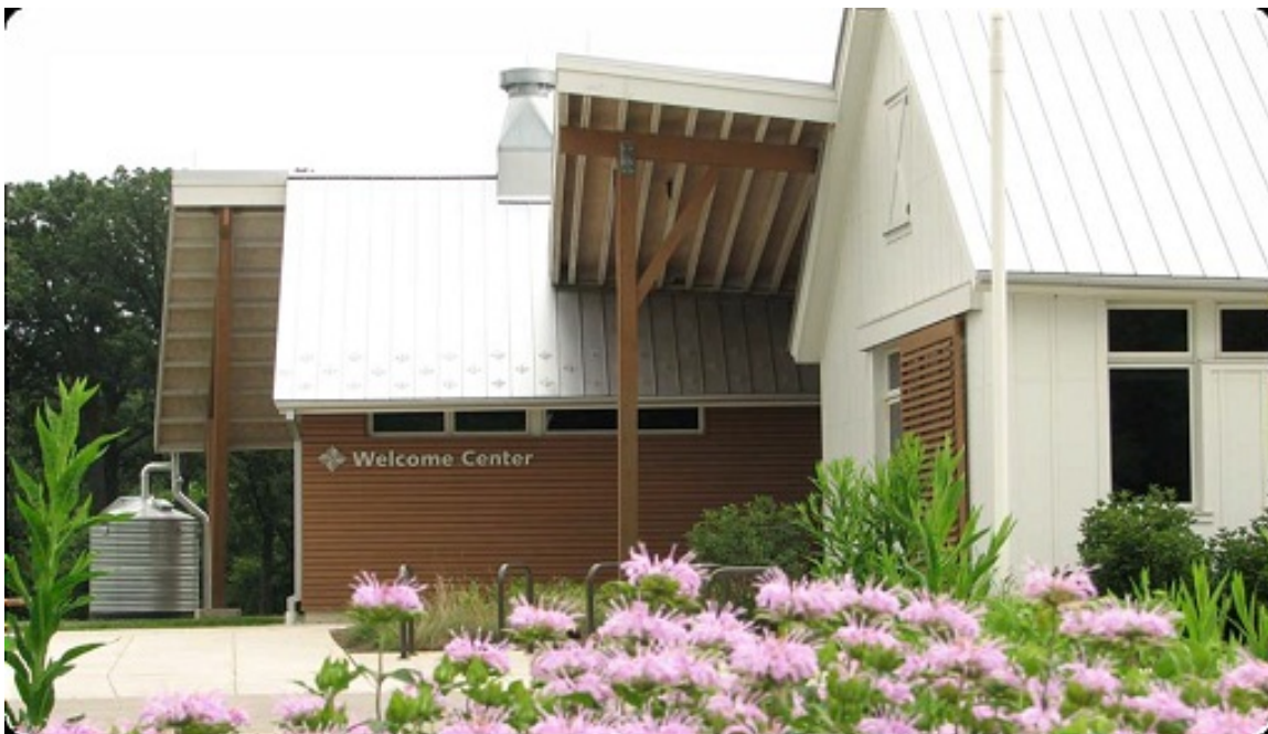
Figure 11.33: A Rain Barrel Collection System This "green" building (Ryerson Woods Welcome Center, Lake County (Illinois) Forest Preserve District) uses both a rain barrel to collect stormwater draining from the roof, and a rain garden to help infiltrate precipitation. Source: Jaffe, M., et al. (2010) (p. 587), Fig. 12, p. 116.
