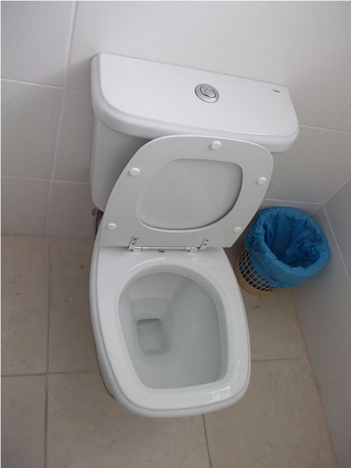
Figure 11.15: Dual-flush Toilet This toilet has two flush controls on the water tank. Pushing only the circular button releases half as much (0.8 gallons, 3 liters) water as pushing the outer button. Source: By Eugenio Hansen, OFS (Own work) [CC-BY-SA-3.0 46 ], via Wikimedia Commons 47 Available for free at Connexions < http://legacy.cnx.org/content/col11325/1.43 >
