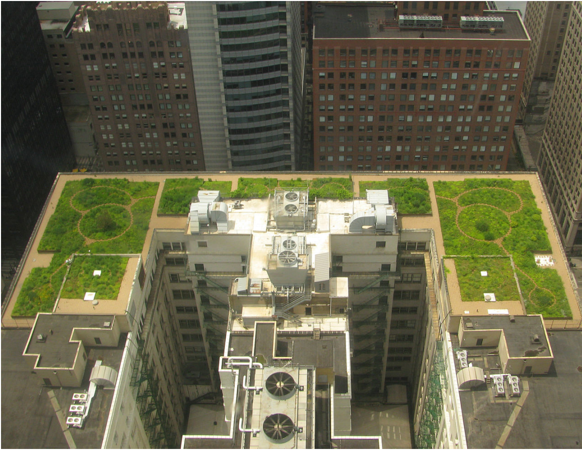
Figure 11.4: Green Roof The green roof of City Hall in Chicago, Illinois Source: TonyTheTiger [CC-BY-SA-3.0 15 ] via Wikimedia Commons 16
