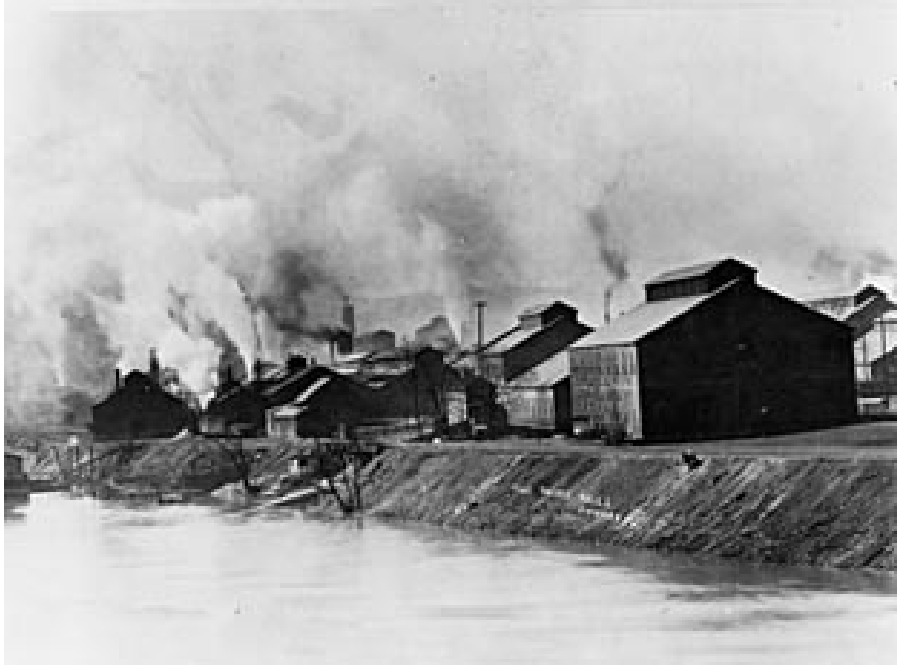
Figure 2.7: Zinc Smelter. Photograph shows a local smelter in a small valley town in Pennsylvania with, essentially, uncontrolled emissions. Source: The Wire Mill, Donora, PA, taken by Bruce Dresbach in 1910. Retrieved from the Library of Congress 63
