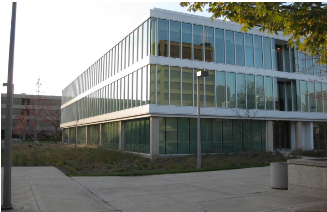
Figure 11.25: Lincoln Hall, LEED Gold Certified, University of Illinois at Chicago Lincoln Hall, LEED Gold certified building on the University of Illinois at Chicago campus. Features include geothermal heating and cooling, solar photovoltaic rooftop system, low-emittance, high-U windows, daylighting, native planting, bioswales for stormwater management, and use of recycled materials. Source: UIC Office of Sustainability 88
