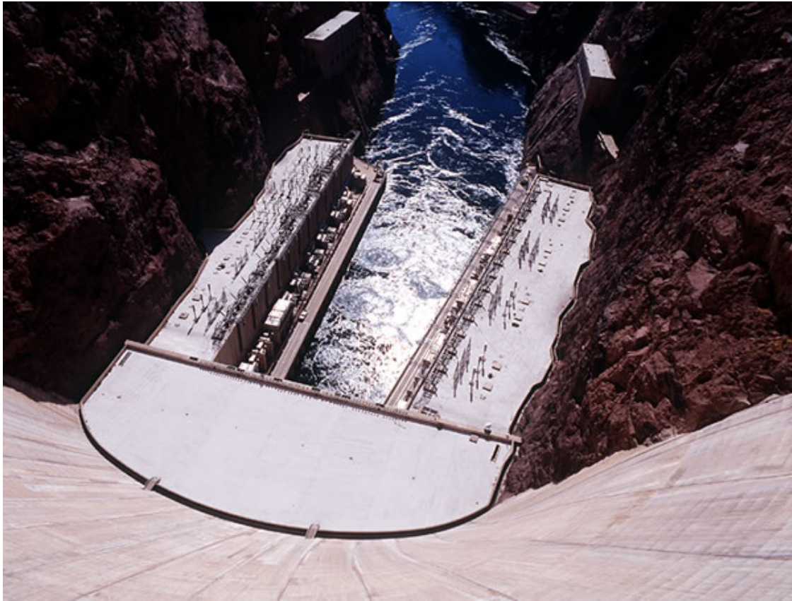
Figure 8.14: Hoover Power Plant View of Hoover Power Plant on the Colorado River as seen from above. Source: U.S. Department of the Interior 41
