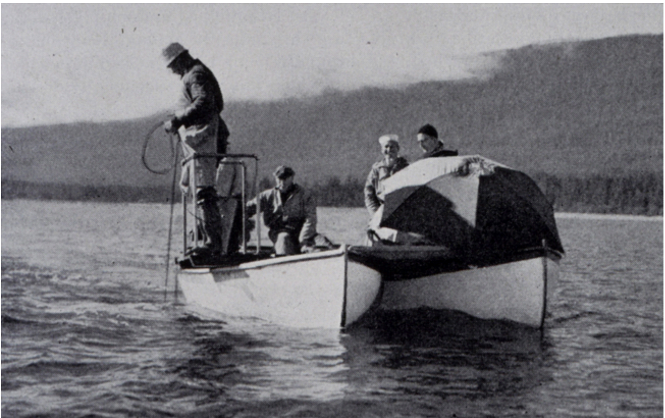
Figure 1.4.1 Lead line survey from a catamaran hull in Alaska, 1942 ( http://celebrating200years.noaa.gov/transformations/hydrography/image7.html ).
