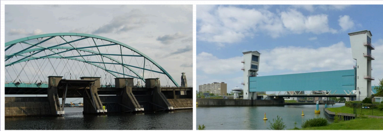
Figure 8.4.6 The Fox Point Hurricane Barrier in Providence, RI, USA (left) and the surge barrier on the Hollandse IJssel river in southern Holland. (Fox Point by Marcbela (Marc N. Belanger) (Own work) [Public domain], via Wikimedia Commons; Dutch barrier by Mark Voorendt (Own work) [CC BY-SA 4.0], via Wikimedia Commons).
