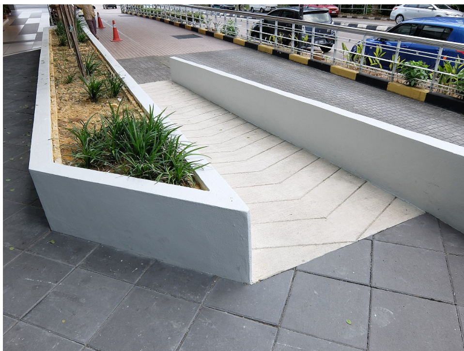
Figure 5.4.7: Pelangi Tower - Wheelchair Ramp | Photograph by Chongian
