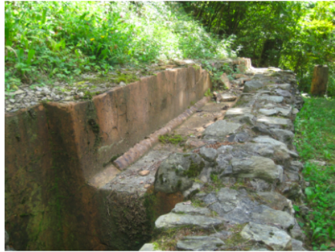
Figure 1.2.4: A section of ancient Roman aqueduct | "Aqueduc romain du Mont Chemin" by Sylenius
