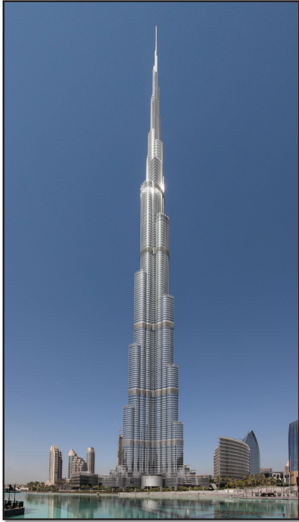
Figure 9.7a | Burj Khalifa, Dubai, United Arab Emirates
