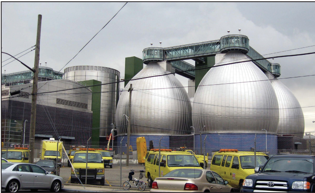
Figure 13.3 | Egg-shaped “digesters” at the Newton Creek Wastewater Treatment Plant
