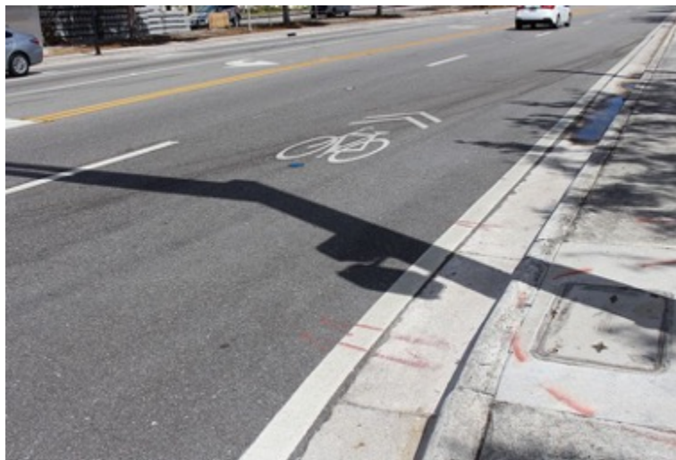
Figure 3.1: Sharrow on US1 in West Palm Beach by Michael Rivera is under the following Creative Commons license: CC BY-SA 4.0
