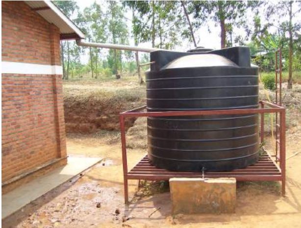
Figure 4.14: Rainwater harvesting storage tank example.
