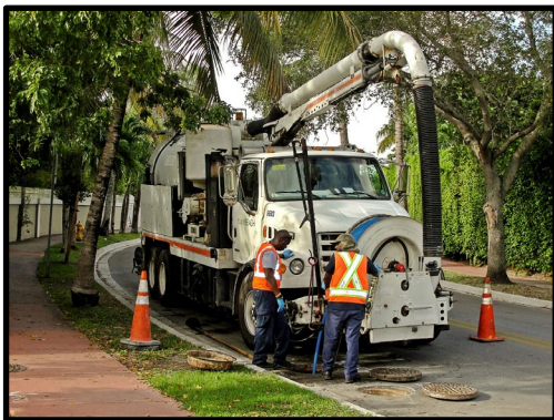
Sewer workers. Beautiful-moments. Used under Pixabay license. https://pixabay.com/photos/construction-workers-manhole-repair-2753799/
