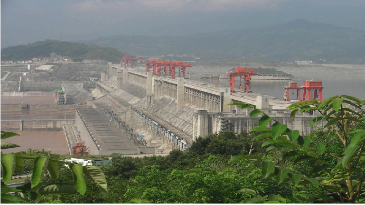
Figure 14.9. The recently completed Three Gorges project on the Yangtze River in China. It is the largest hydroelectric facility in the world.
